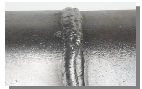
Final weld after several beads are made
